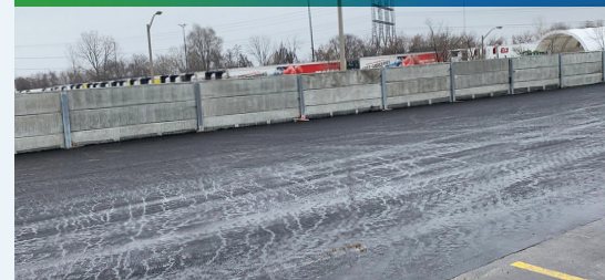
Completed wall installation
