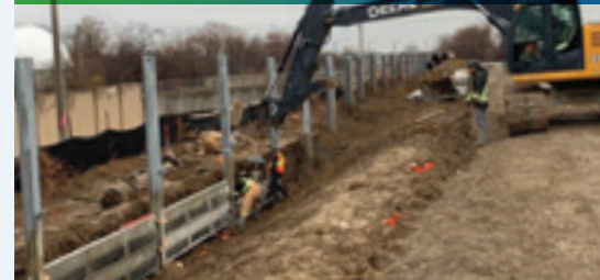
Installation of lower MSE earth retaining wall panels
