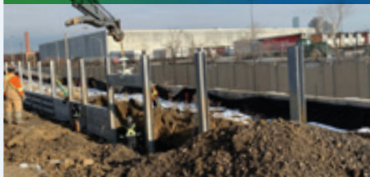
Installation of lower MSE panels and lower panels
