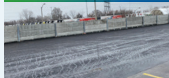
Completed wall installation
